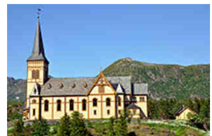
Lofotenkathedrale in Kabelvåg
